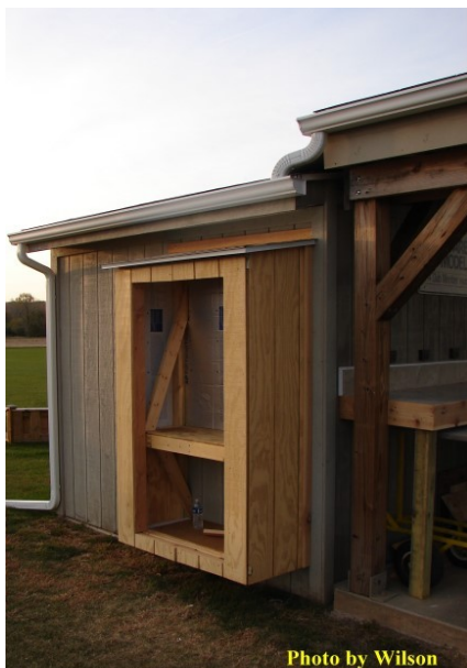
Here is the generator cabinet under construction.
