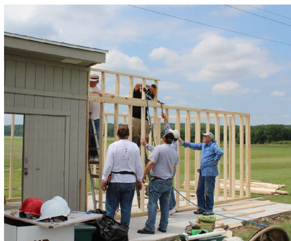
PRCM's highly skilled work crew begins framing up the shed extension.
